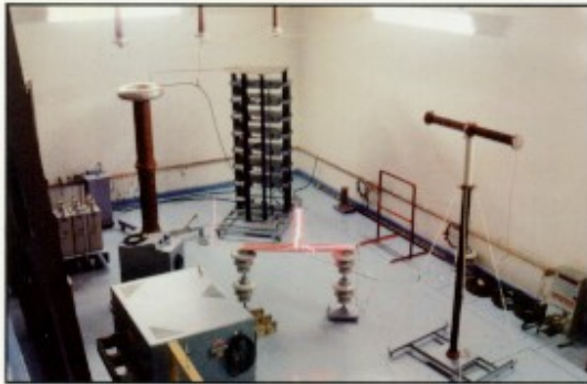
400kV impulse Test on Standoff Insulator and Insulated Bus using 700kV Generator.
