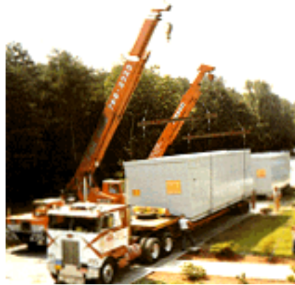
Climatized 13.8kV Metal-Clad for Petrochemical Plant
